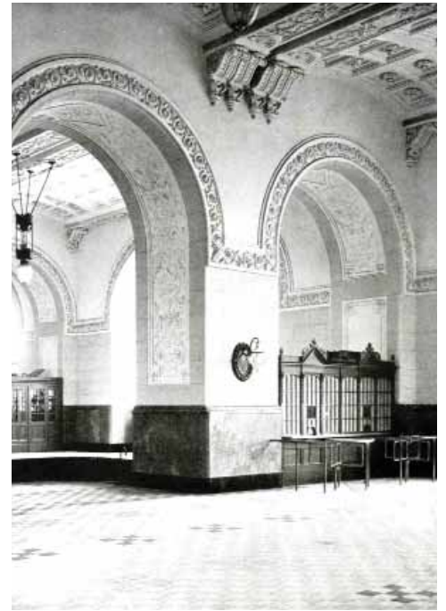
Haydar Paşa Station
